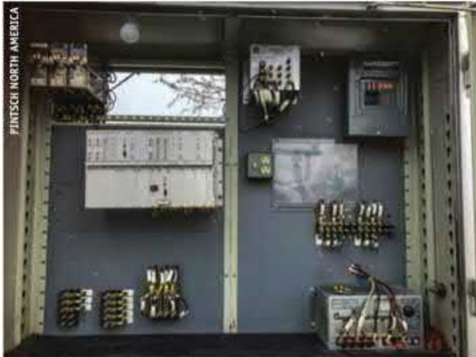
This image shows an old relay case reconfigured by Pintsch with new train detection technology.
